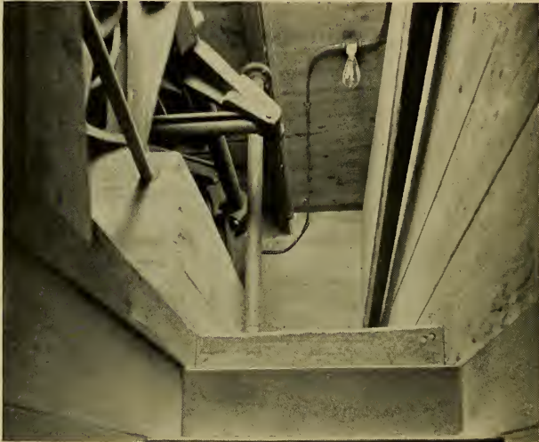
Fig. 155—Entrance Way into the Foundation Pit of a Jolt-Moulding Machine, showing Steps leading into the Pit from an Adjoining Basement Room.
